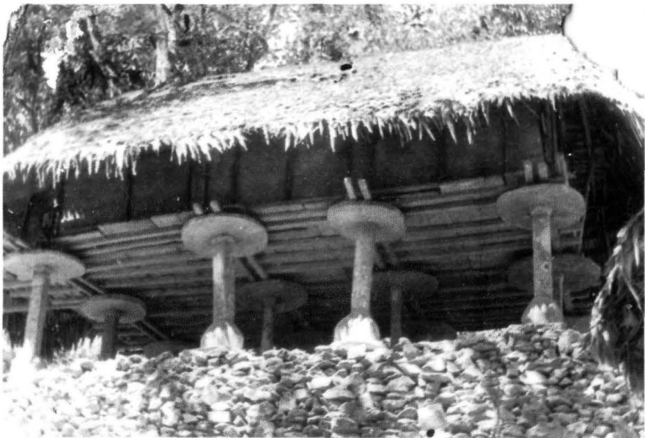
An Adi barn with protection posts for checking entry of rat
